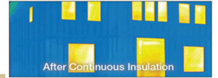
Adding exterior continuous insulation prevents heat flow through framing.
